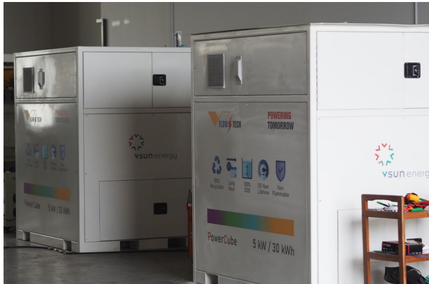
Figure 8: VSUN Energy branded V-Flow Tech 5kW/30kWh VRFBs
