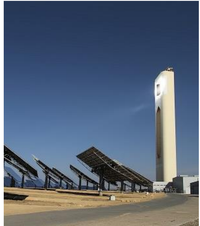
Concentrated Solar Energy Tower with parabolic concentrating mirrors
