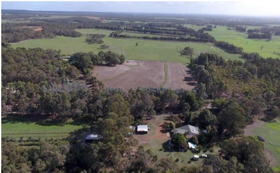
The Busselton property where the battery will be installed
