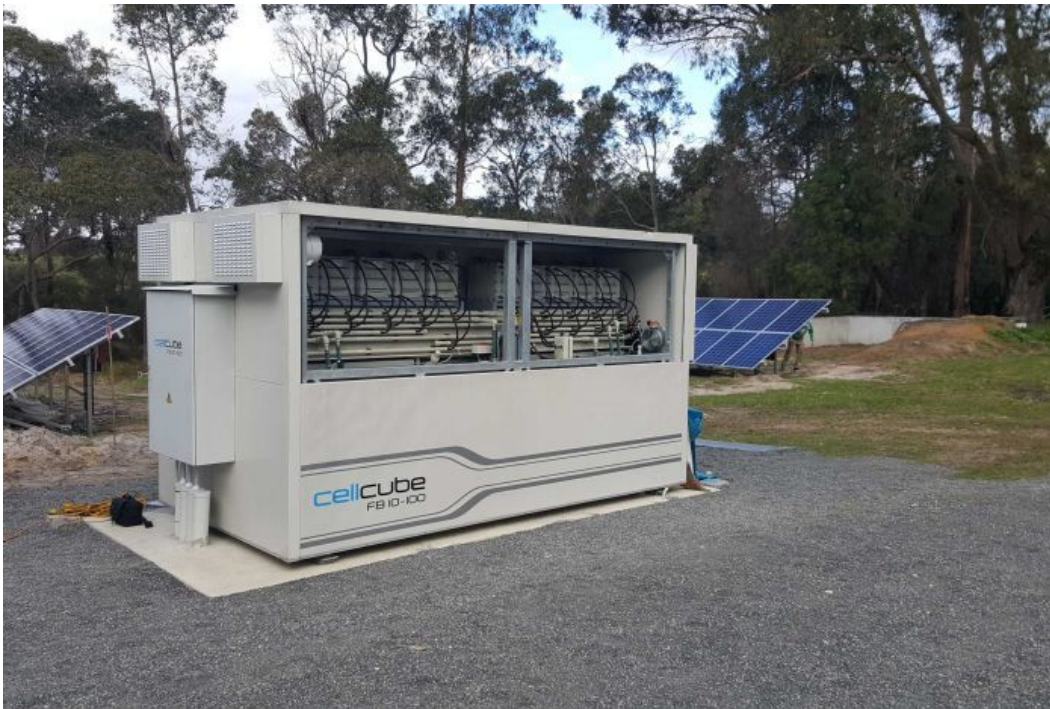
PHOTO: The flow battery, also known as a redox battery, is made with vanadium, a tech metal found in Australia (Supplied: VanadiumAustralia)
